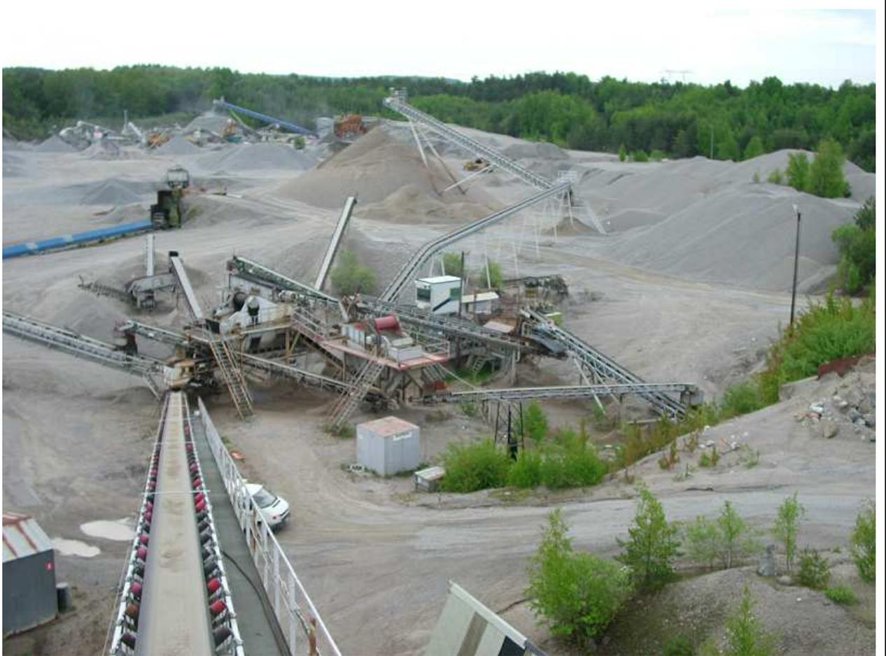
*In the foreground is seen gravel plant and in the background crushed rock plant. Total production is now about 400 000 tons per year. 30 years ago it was about 1 000 000 tons.*
